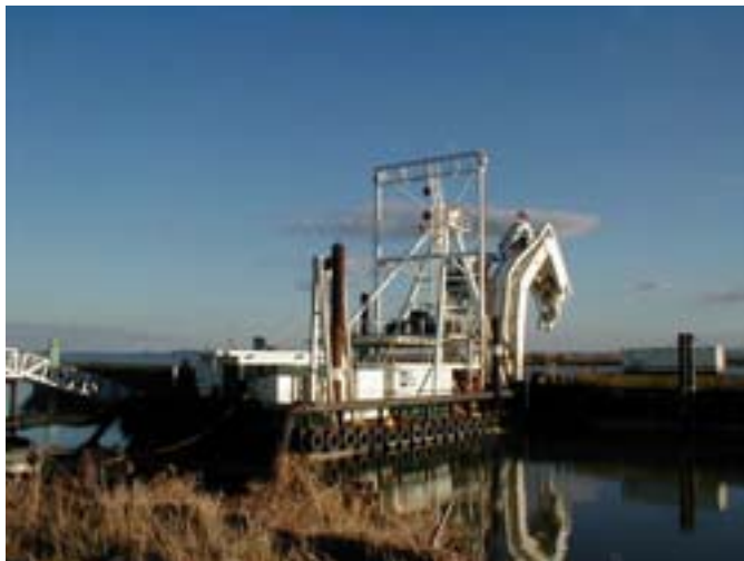
Figure 5-4. Offloader at Hamilton Wetland Site (Photo: USACE)
