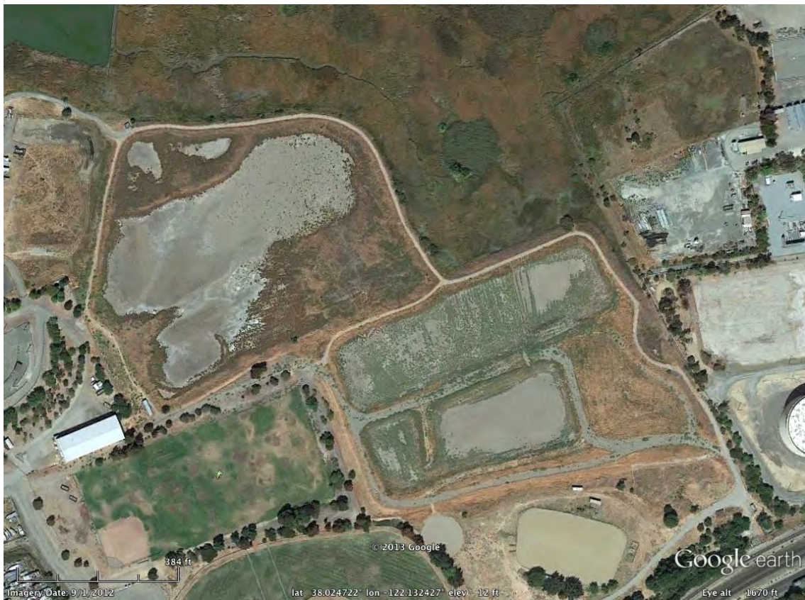
Dredge Materials Storage Ponds at Martinez Marina
