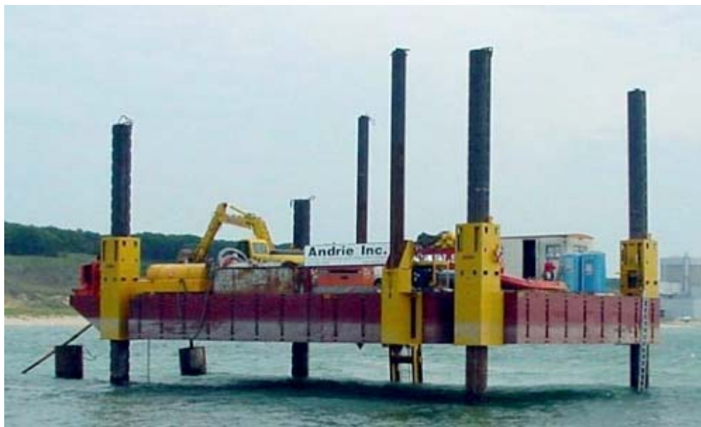
Figure 7-3. Jack-Up Barge. Source: IMC Brokers
